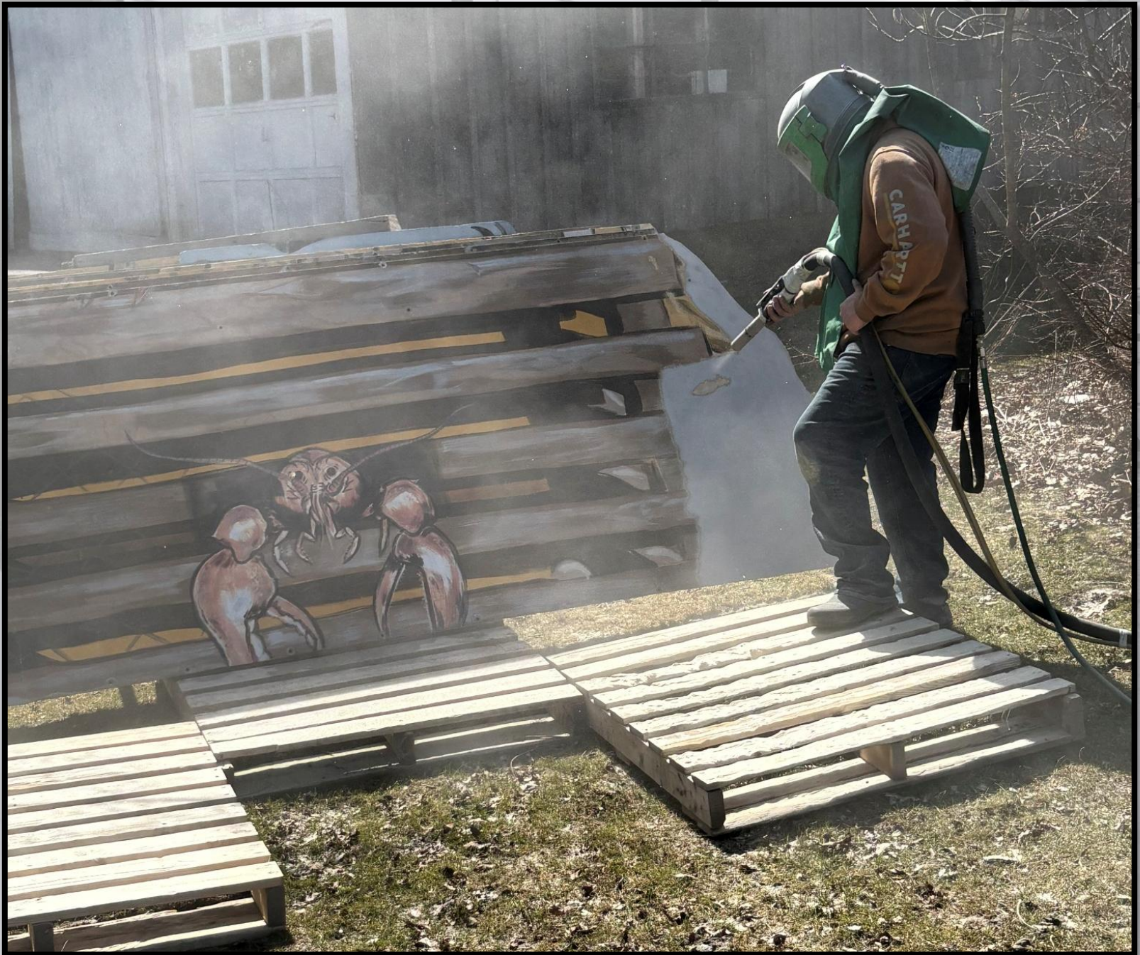
Old paint removed by air-blasting
